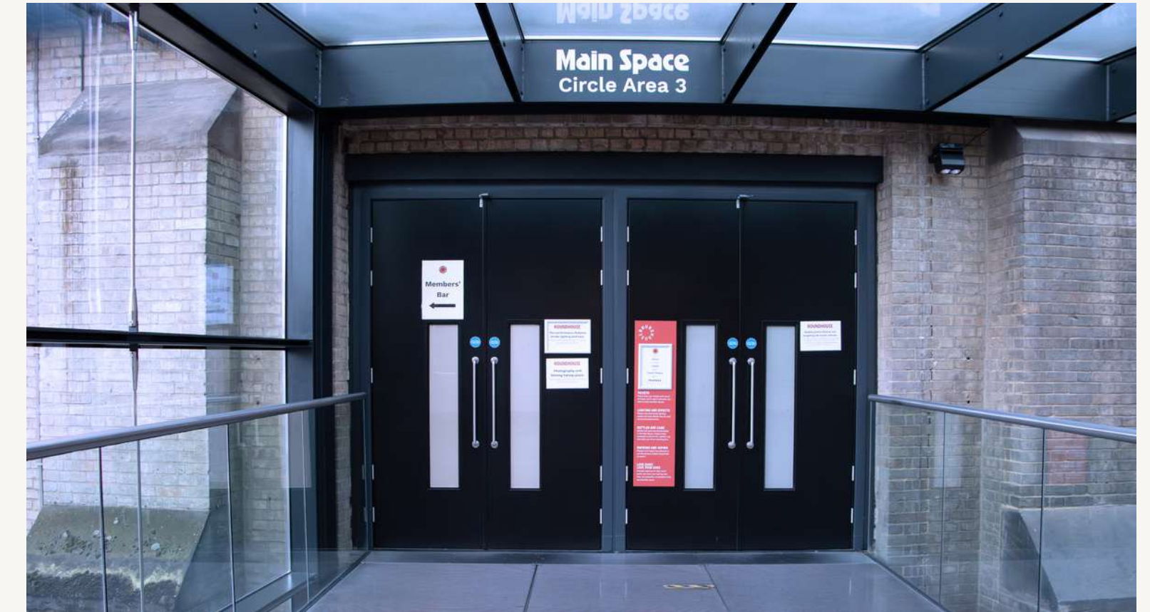
LEVEL 2 DOORS AREA 3
