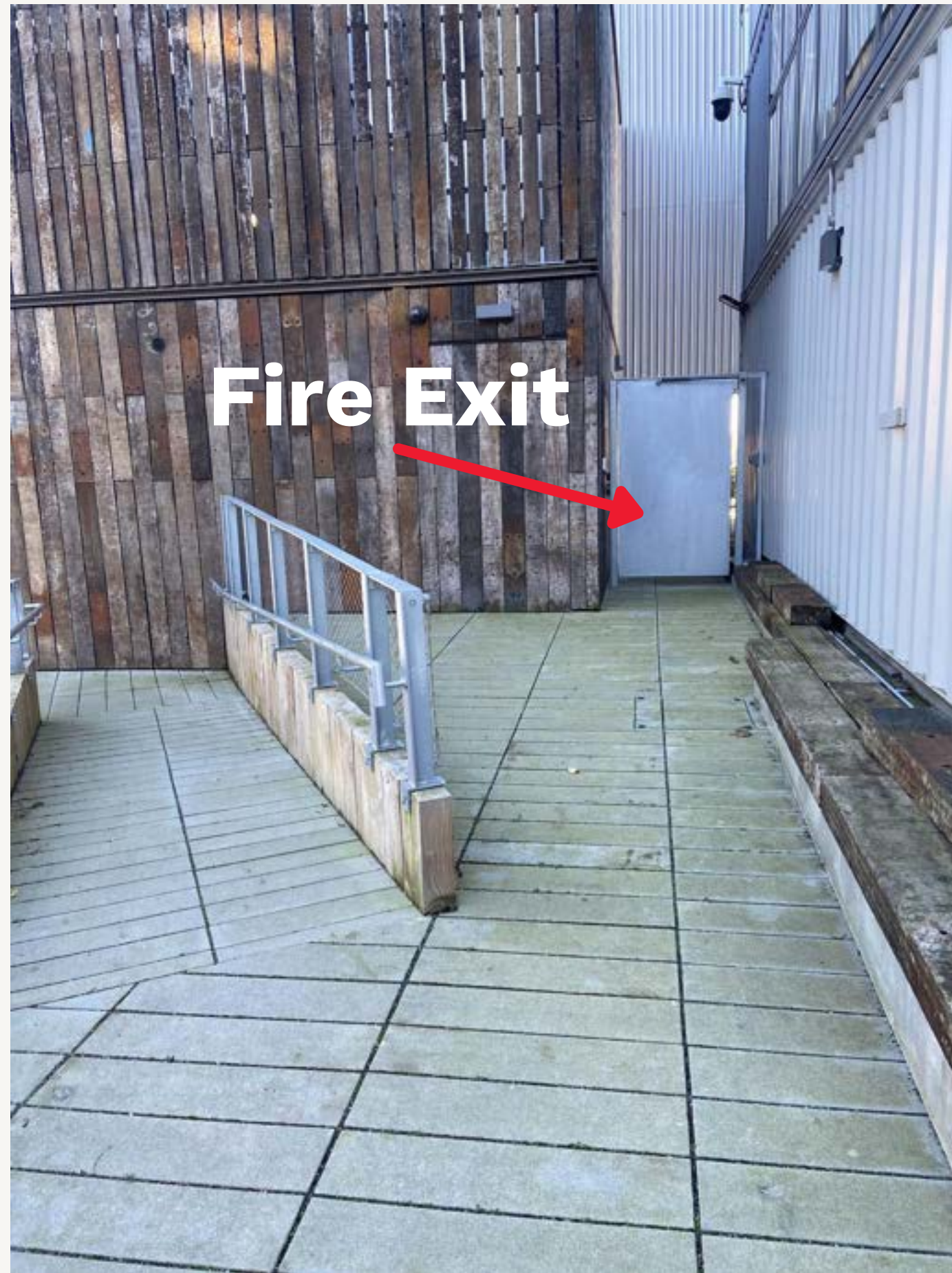
Fire exit on the external ramp
