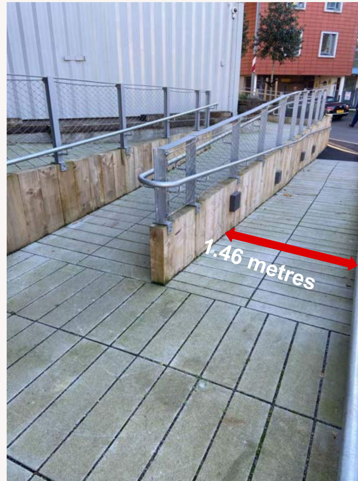
Wide corner bend
