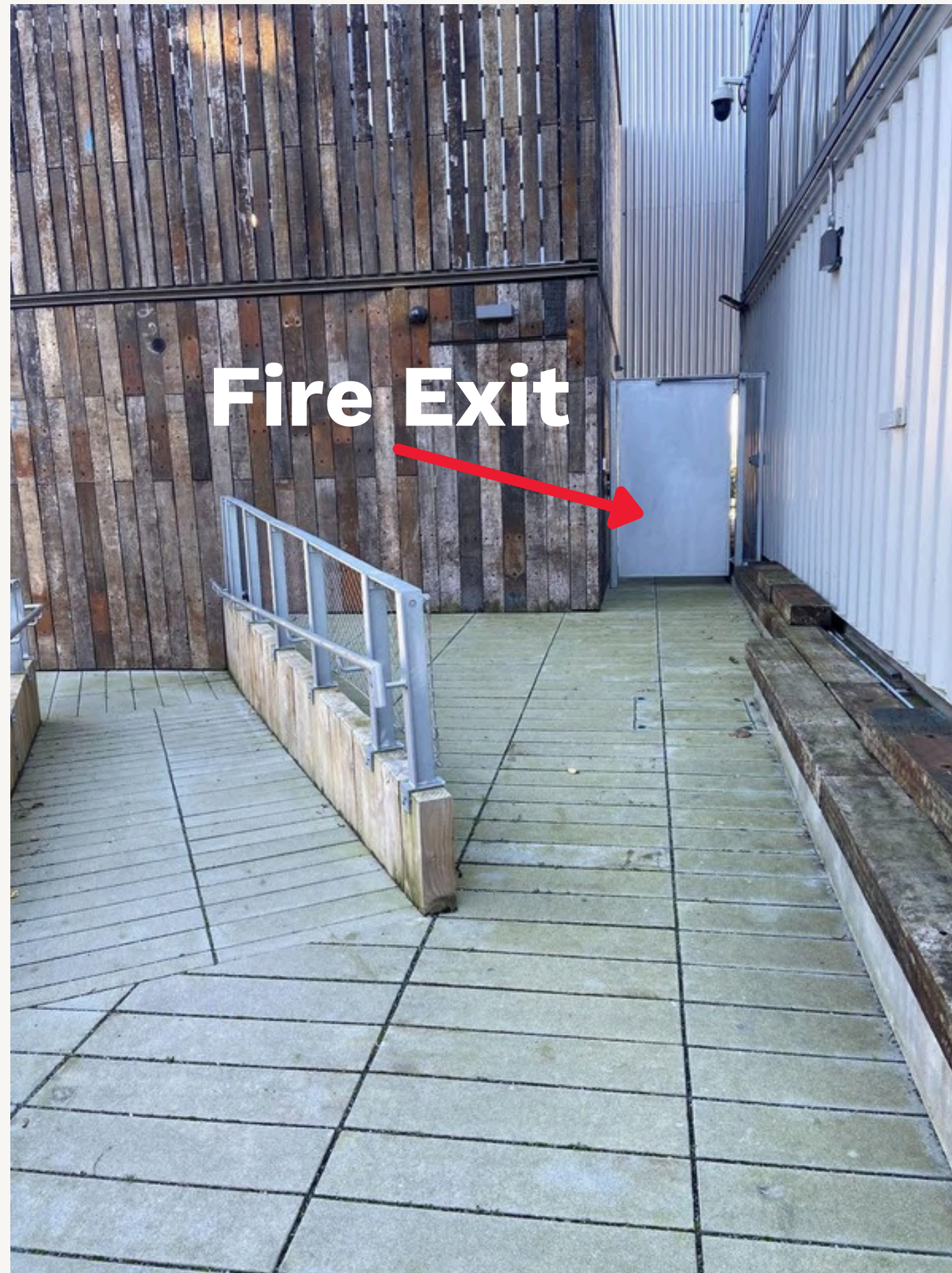
Fire exit on the external ramp
