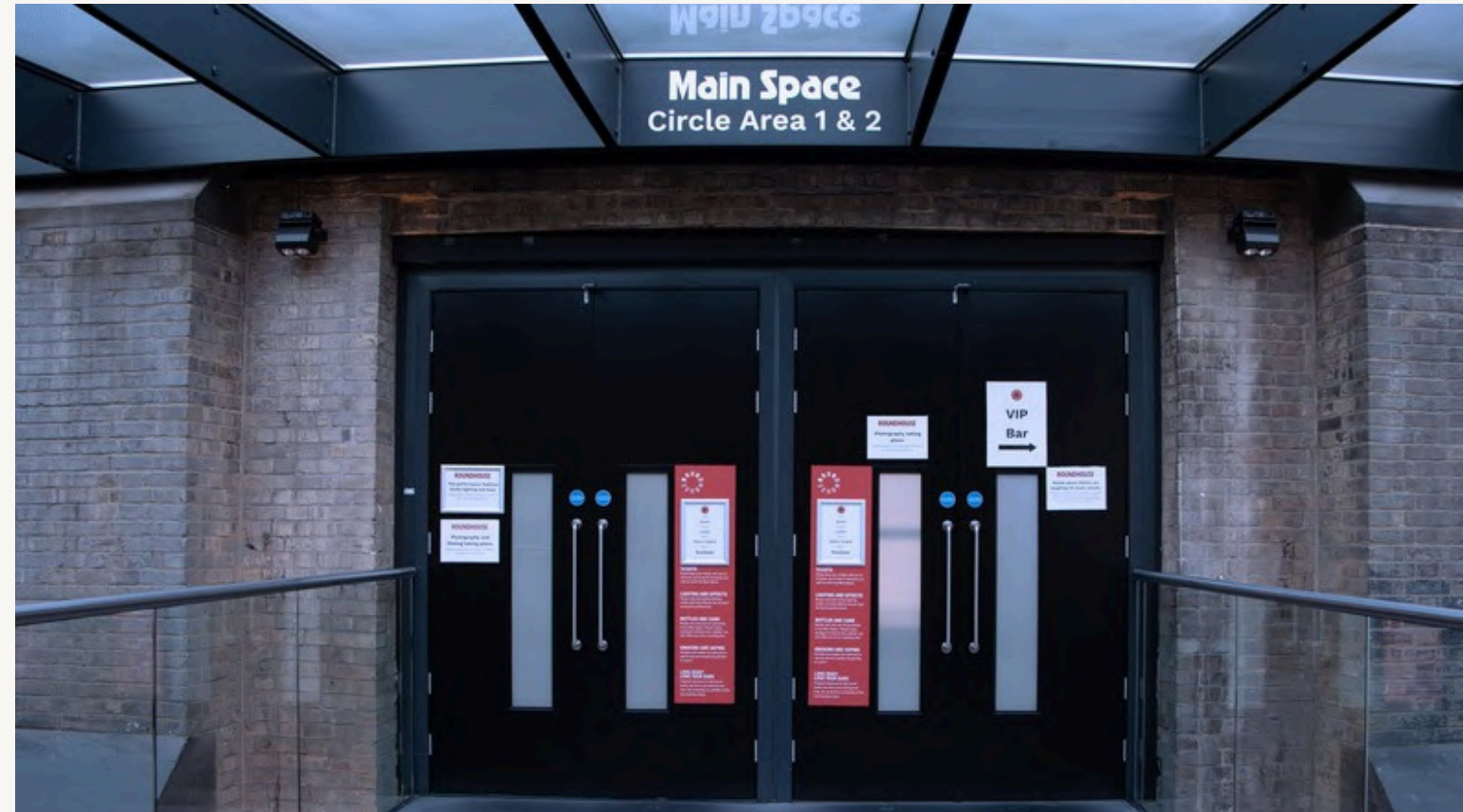
LEVEL 2 DOORS AREA 1&2
